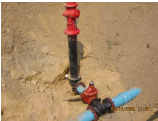
Drain holes are located at the base of the hydrant
